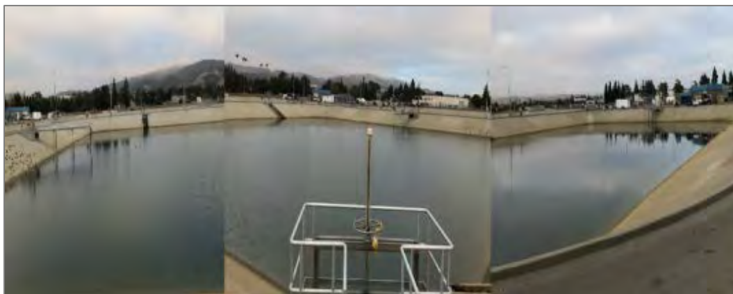
Storage basins in full capacity after dewatering of pipeline
