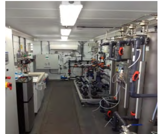
Xylem MiPro containerized O3/BAF and UV AOP system
