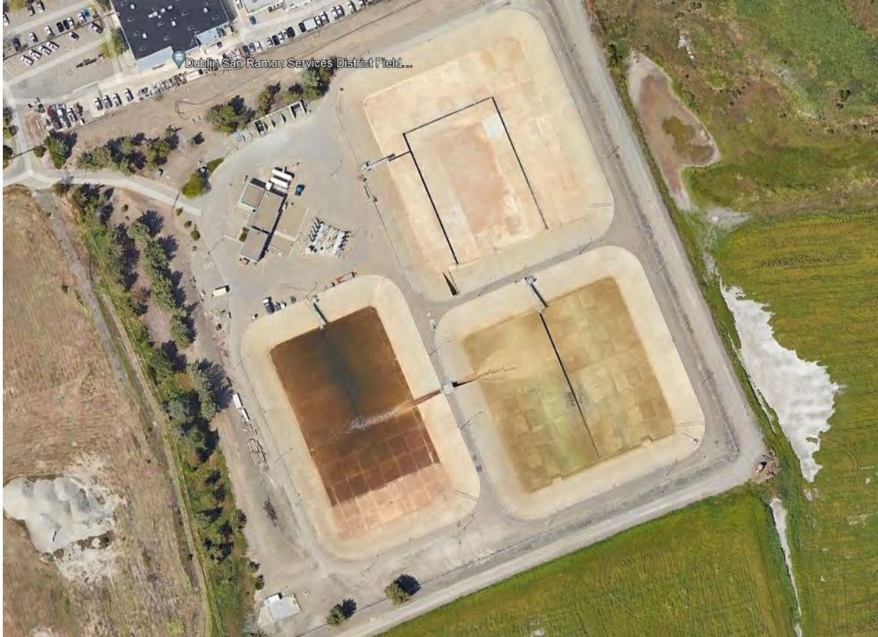
Photo 3 – Aerial View of Pump Station
