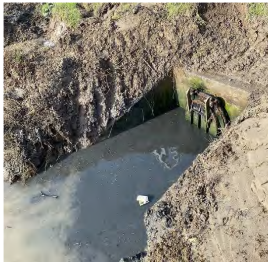
Photos: Before and after photos of the discharge point that was cleared of soil and silt runoff from the January 2023 storms.
