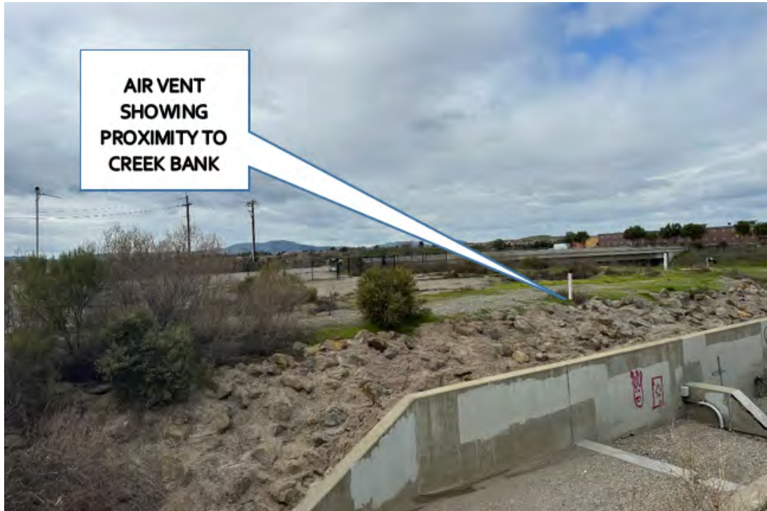
Photo 1.4: Parallel Creek Embankment Risks
