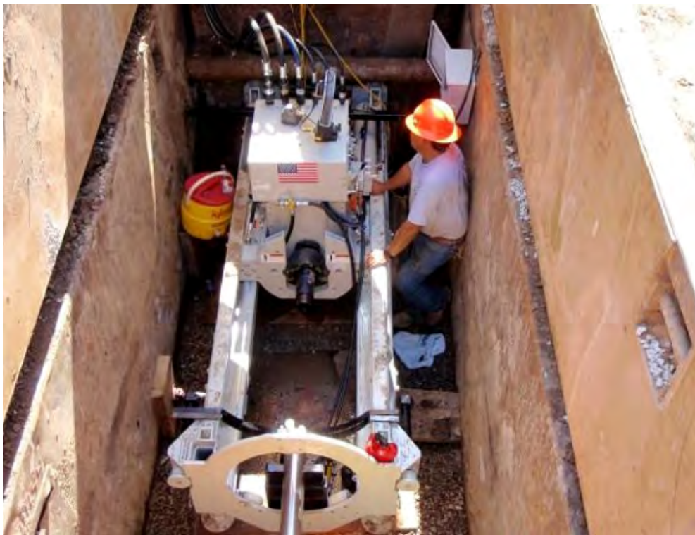
Photo 1.14: Example Auger Bore and Jack Installation
