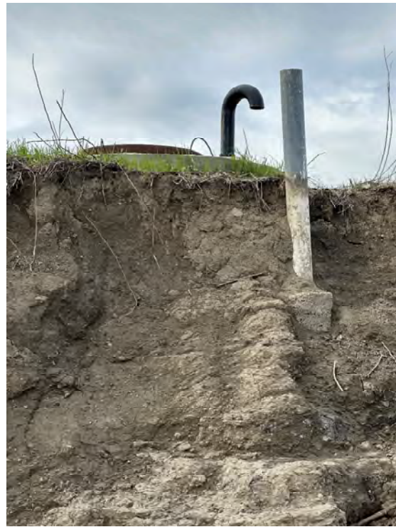
Photo 1.1: Pipe Exposed In Creek Bed (2/14/2023) Photo 1.2: Creek Bank Continuing To Erode (2/14/2023)
