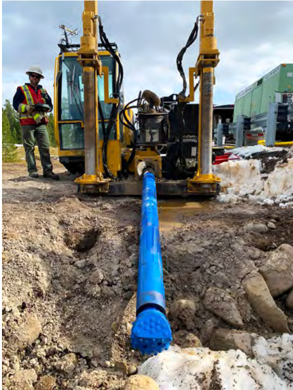
Photo 1.13 Example HDD Installation
