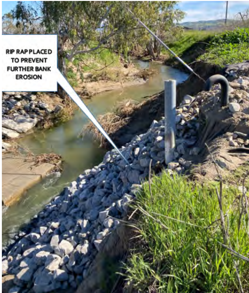
Photo 1.6: Temporary Repair (3/27/2023) Photo 1.7: Temporary Repair (3/27/2023)
