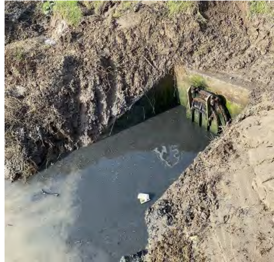
Photos: Before and after photos of the discharge point that was cleared of soil and silt runoff from the January 2023 storms.
