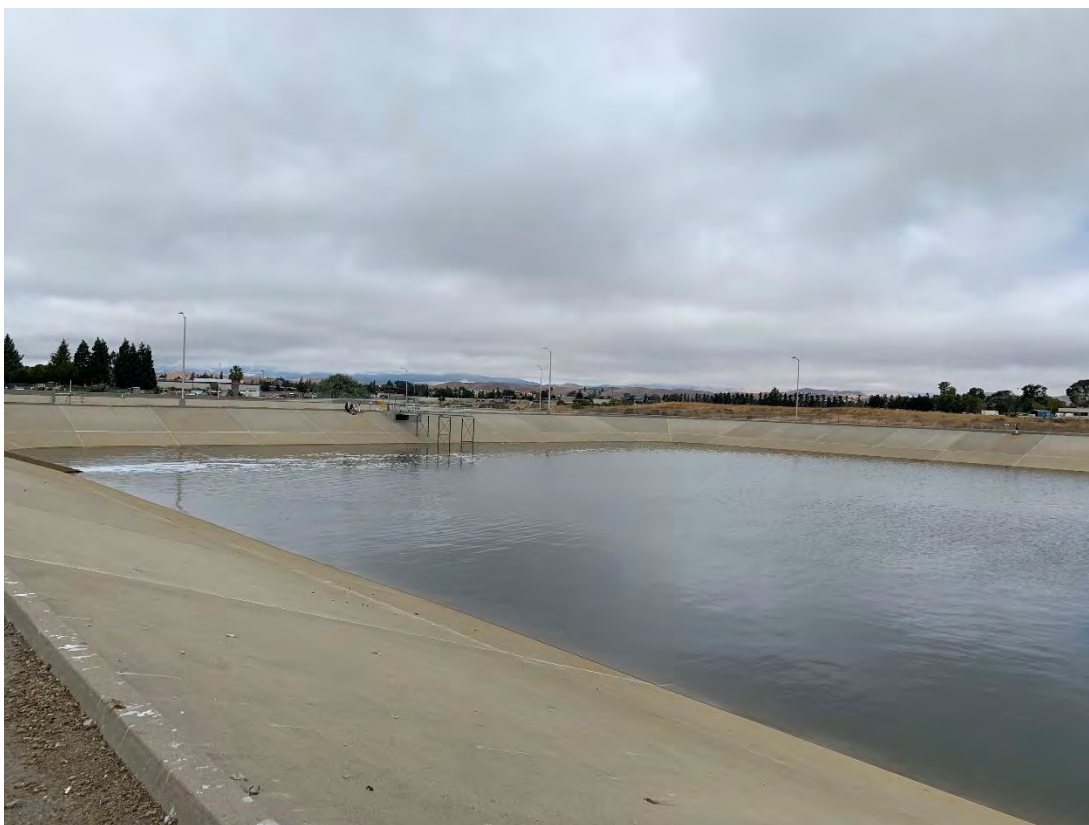
Figure 2. Fully treated wastewater from the City of Livermore and DSRSD treatment plants is combined and then flows through the middle gate (Figure 3), which equalizes wastewater flows between the Facility’s equalization basins.
