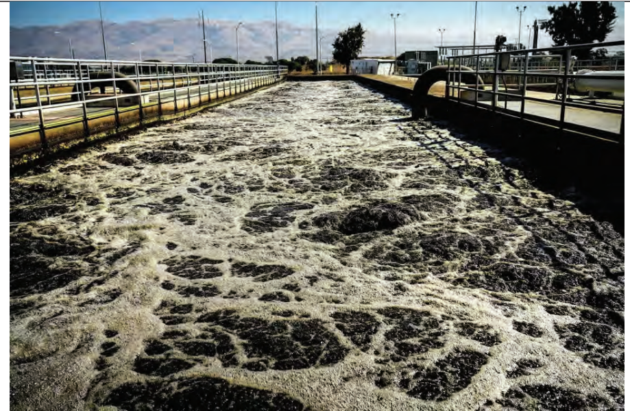
Sewage undergoes biological treatment in a tank at the San Jose-Santa Clara Regional Wastewater Facility in 2022.
