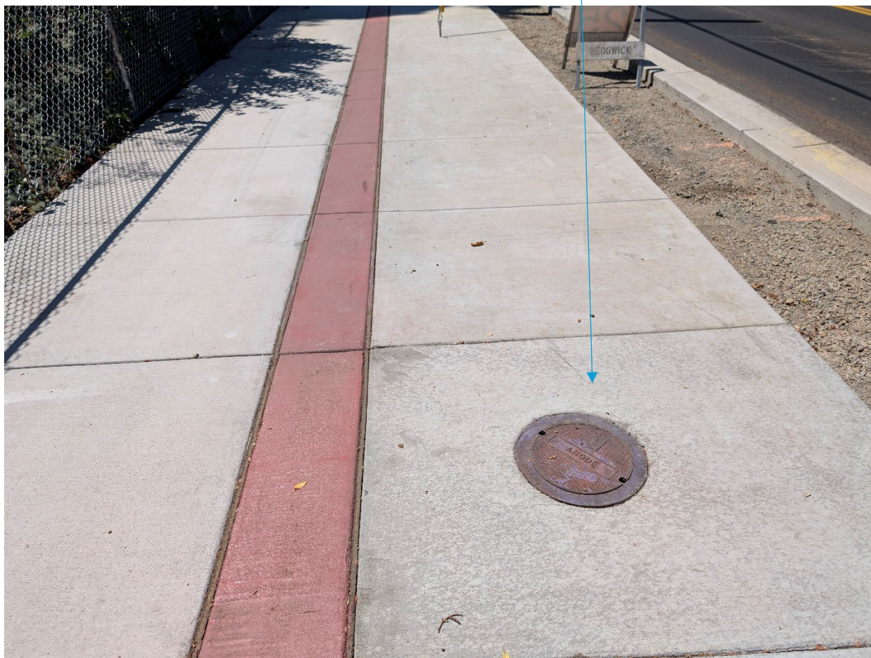
Sidewalk on August 14, 2025 – LAVWMA Cathodic Test Station (after)
