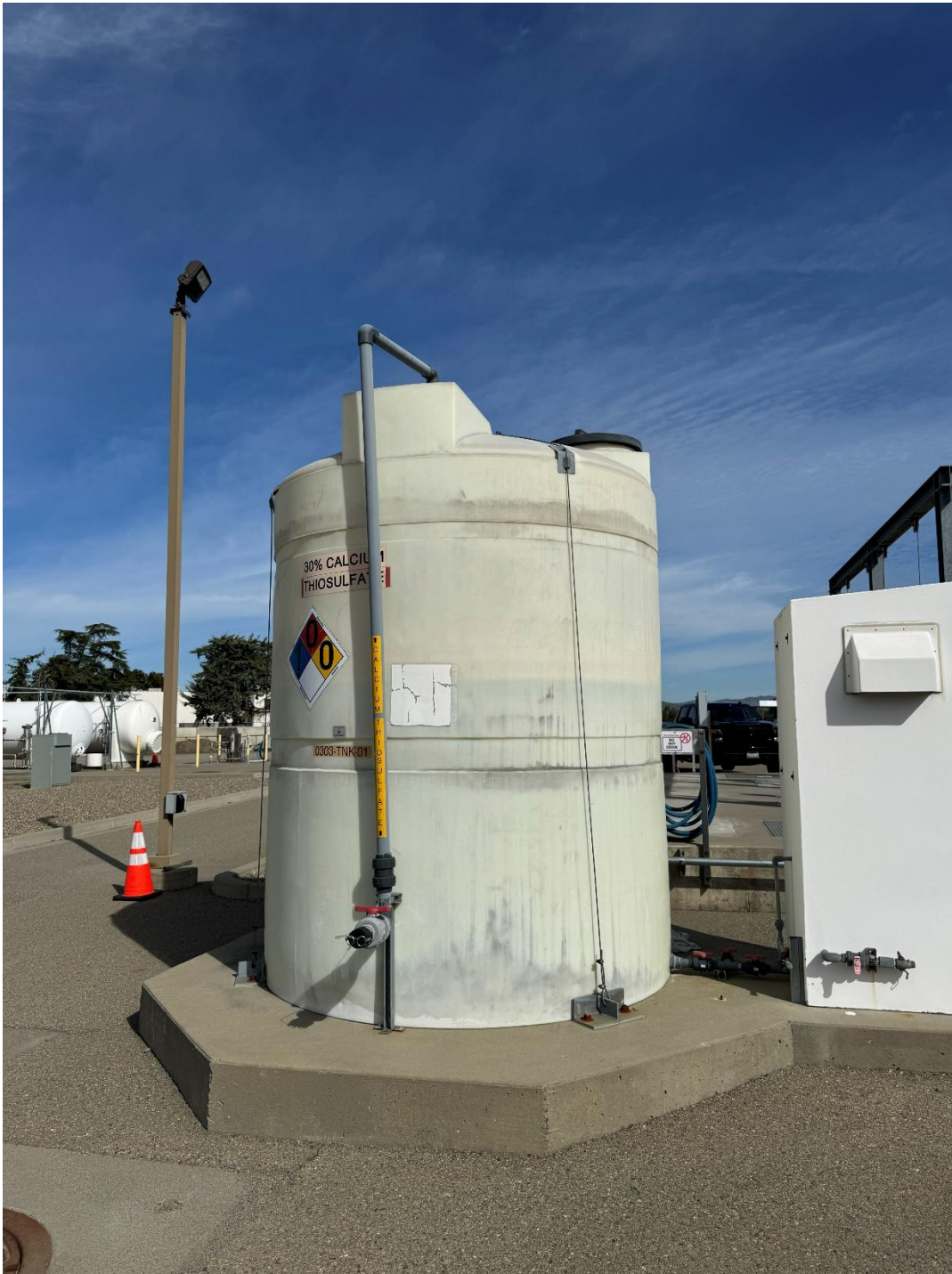
Figure 4. Calcium thiosulfate, used for dechlorinating wastewater during wet weather discharges or discharge exercises.
