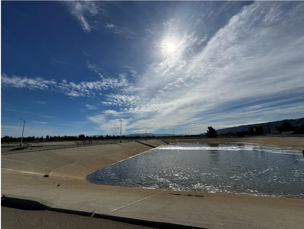
Figure 3. One of three holding basins on site. Fully treated wastewater from the City of Livermore and DSRSD treatment plants is combined and then flows through the middle gate, which equalizes wastewater flows between the Facility's equalization basins.
